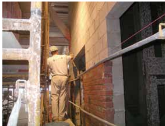
Guardrails protect employees from a fall hazard, nice job
