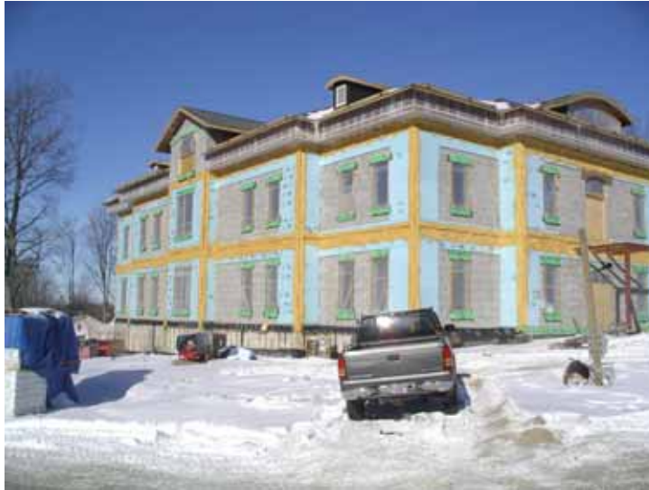
The job at Hillsdale is ready for veneer
