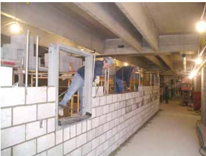
Jim Varga works around a window frame at Oakwood Hospital
