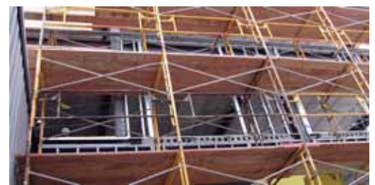
Scaffold at Sparrow Foster Wing in Lansing, MI
